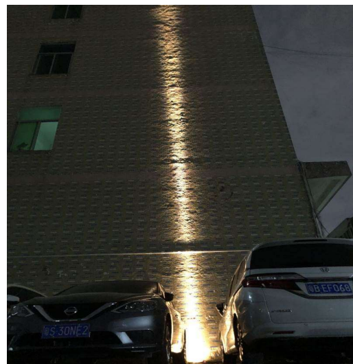
With 9Watt led, result of wall-washing
